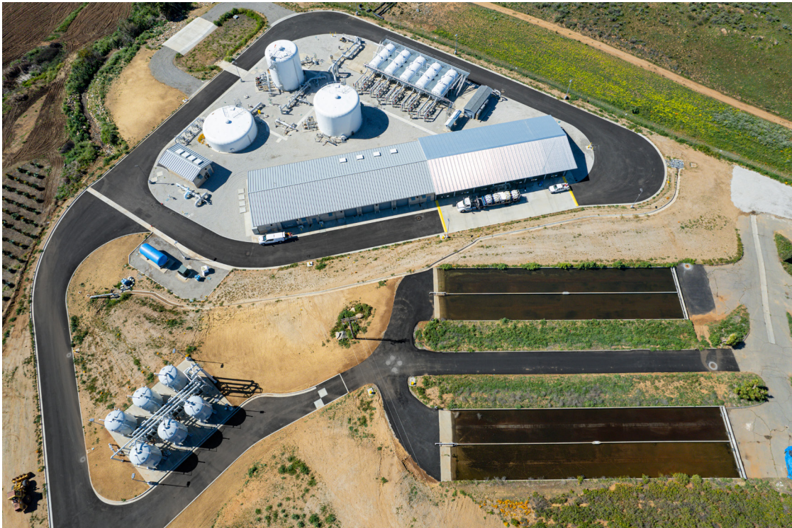
Santa Margarita Groundwater Treatment Plant
