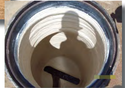
Pipeline relining program
