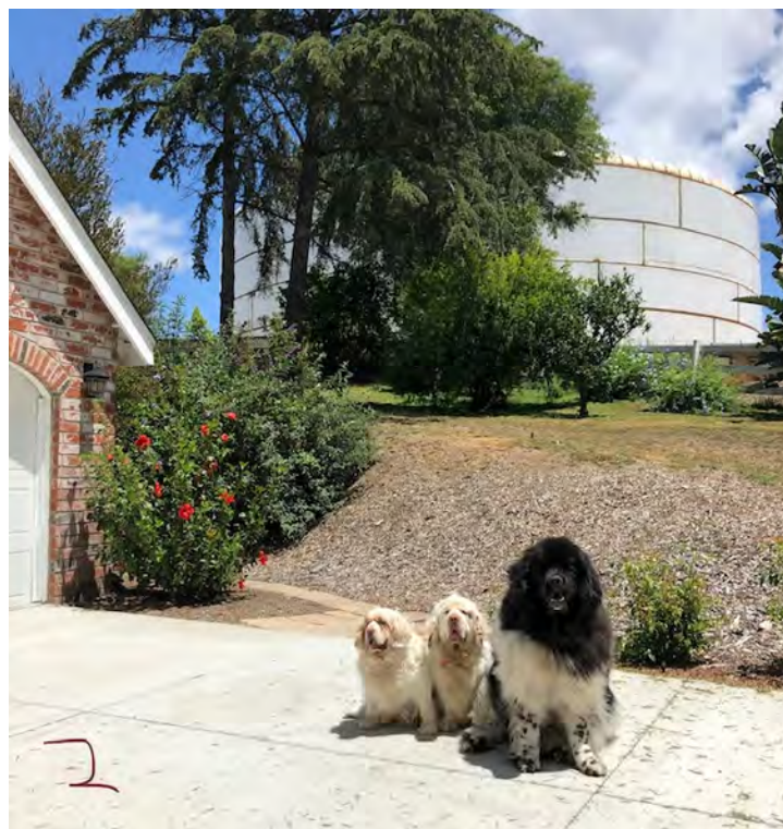
New Tank Driveway View
