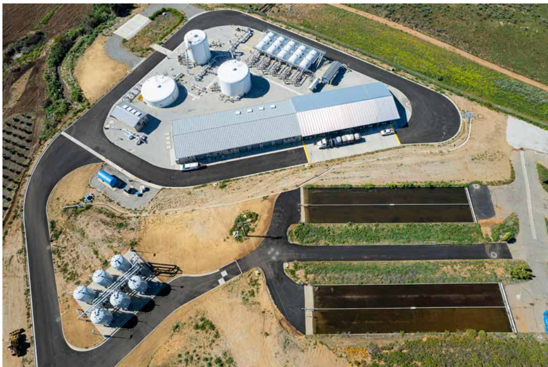
Santa Margarita Groundwater Treatment Plant
