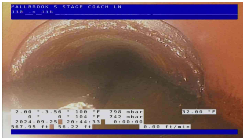
COL-P2PZ-GSMN-J38-J36_70bbd1a3-fd2b-4296-bc17-9d303d25b5c9_20240925_115601_248.jpg, 00:03:24, 56.22ft Joint Offset Medium
