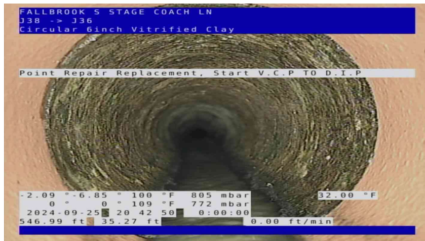
COL-P2PZ-GSMN-J38-J36_23aebbc7-0c66-4c7f-a22b-586c9cdc2145_20240925_115418_06 2.jpg, 00:01:58, 35.27ft Point Repair Replacement, Start / V.C.P TO D.I.P
