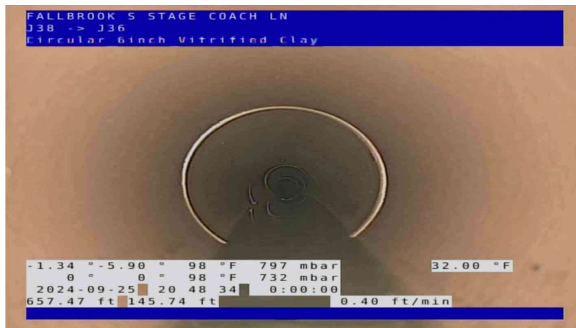
COL-P2PZ-GSMN-J38-J36_db9685e3-6cdb-4b8d-a2a6-d1e8b8504aab_20240925_120001_911.jpg, 00:06:52, 145.74ft Miscellaneous Water Level, Sag, 20% of the vertical dimension, Start
