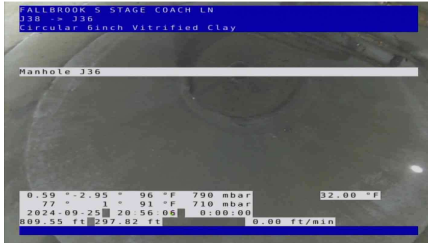
COL-P2PZ-GSMN-J38-J36_8371e5b5-6237-48eb-9a16-521a20883ec2_20240925_120733_402.jpg, 00:12:56, 297.82ft Manhole / J36
