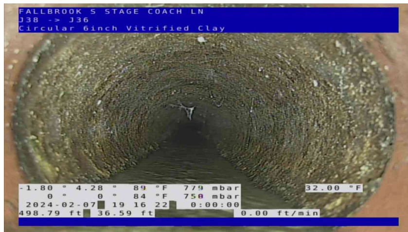
COL-P2PZ-GSMN-J38-J36_53f5c61a-9842-45c2-ba0b-f57b332dc318_20240207_092457_121.jpg, 00:04:05, 36.59ft Miscellaneous Material Change / VCP TO DIP
