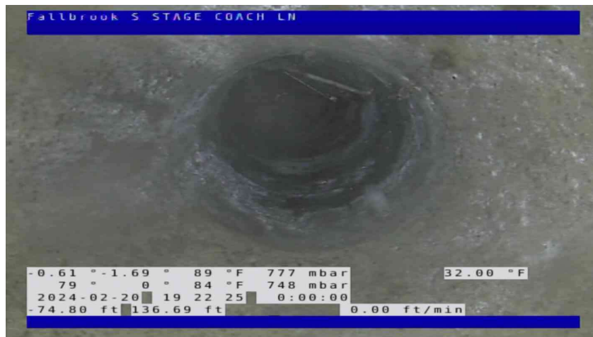
COL-P2PZ-GSMN-J12-J10_7ff1b602-baf4-4975-80a2-10ba69e419ad_20240220_093113_282.jpg, 00:03:18, 136.69ft Manhole / J10
